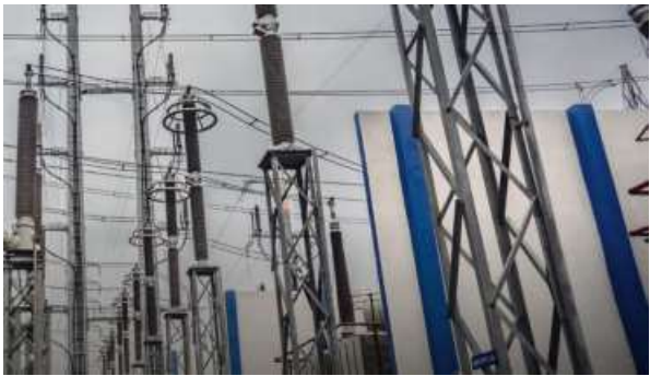
POWERING AHEAD. Godrej is building a 400 kV gas-insulated switchgear substation with a 1.2 GW stabiliser, and a 765 kV GIS bay extension to strengthen Gujarat's transmission network
